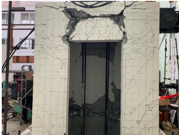
现浇电梯井筒破坏形态
